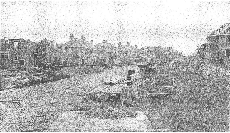
Chandos Road under construction in 1932. (Photograph courtesy Messrs Cadbury's Ltd.)
